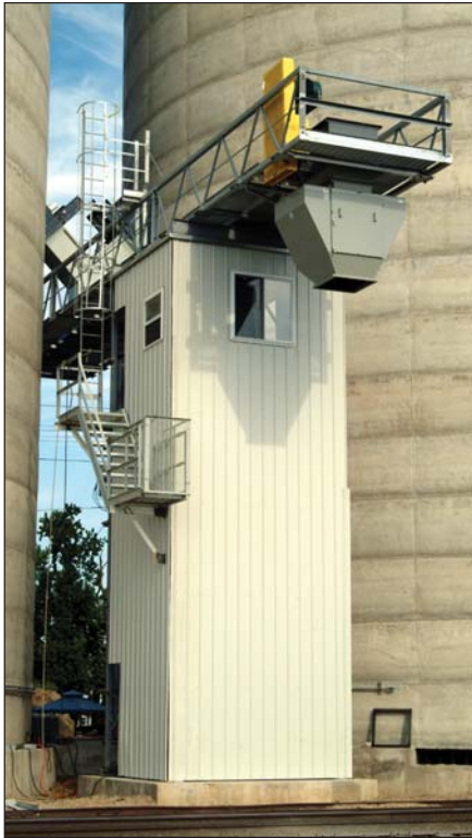
Two-story loadout shed, with a 40,000-bph Union Iron Works loadout drag conveyor and spout.
