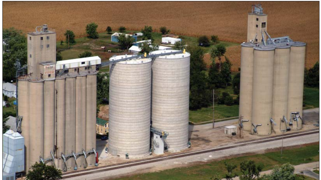
Ludlow Coop Elevator Co.'s flagship elevator in Ludlow, IL, with two new Hoffmann jumpform concrete tanks at the center of photo. Aerial photo by B&M Studio of Photography, Pekin, IL.
