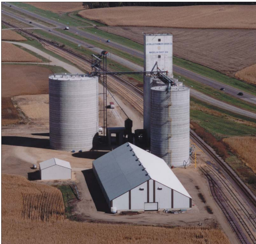
LaSalle Farmers Grain Co.'s rail terminal near Madelia, MN, including a new 700,000-bushel Hoffmann jumpform concrete tank on the left side of the facility. Photo courtesy of Hoffmann Inc.
