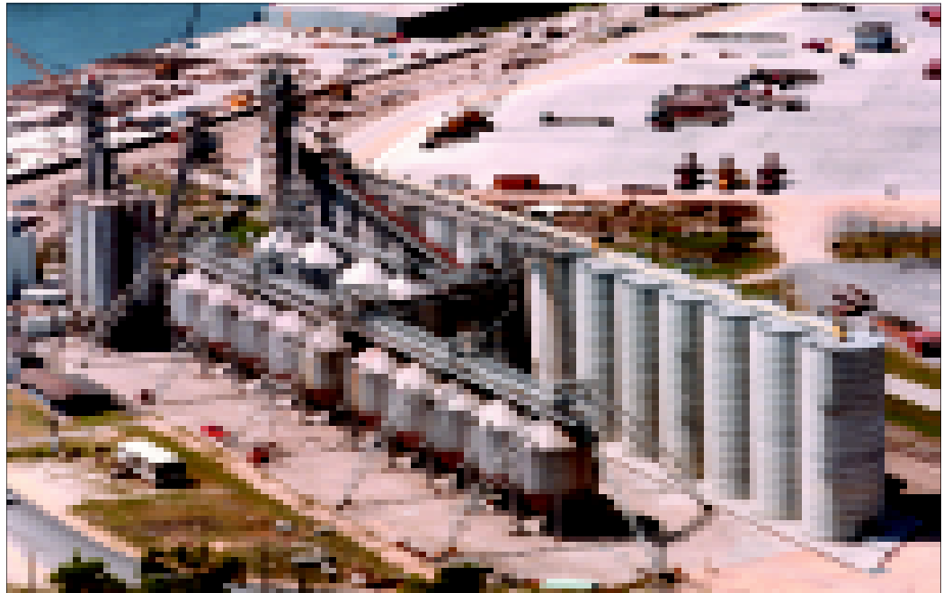
Grain elevator serving the Lake Charles Harbor & Terminal District in Lake Charles, LA. New six-tank, 270,000-bushel jumpform concrete annex can be seen at right. Photo courtesy of Hoffmann Inc.
