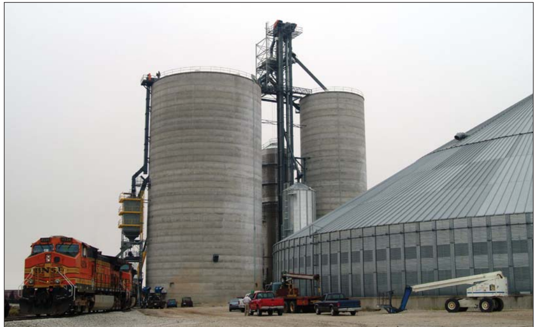
BNSF shuttle train at left awaits loading in mid-September. Photo shows two new Hoffmann jumpform concrete tanks, two Schlagel legs, CompuWeigh bulk weigh loadout system, and Big Chief steel tank constructed in 2001. Ground-level photos by Ed Zdrojewski.
