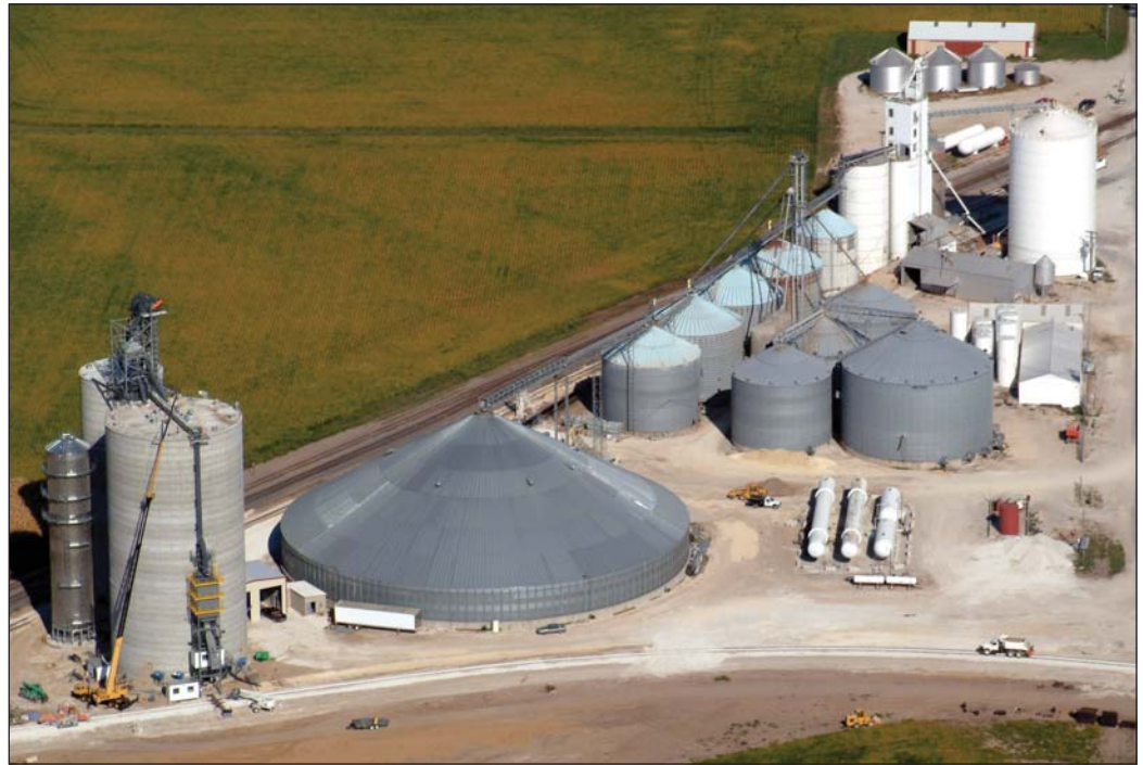
Aerial view of the Farmers Elevator Co. elevator at Lowder, IL, with new rail terminal annex nearing completion at left. Aerial photos by B&M Studio of Photography, Pekin, IL.
